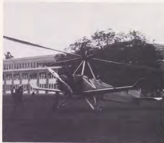
First Pitcairn autogiro, in 1931, had four-bladed rotor, turned-up wings.
