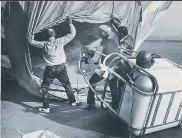
Above—Aids hold the mouth of the partially inflated envelope open while the aeronaut turns on the propane burner to start heating the air. Right, basket assembly is inspected.
