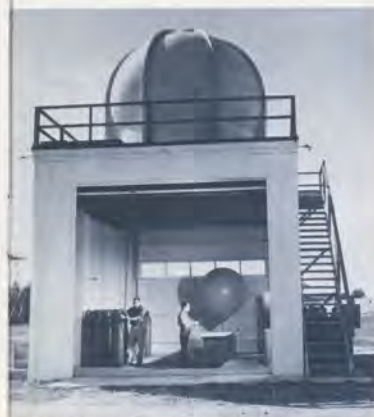
Balloon is filled with gas to lift instruments into upper air to measure temperature, barometric pressure, humidity. Wind direction and speed are computed by tracking radio signals.
