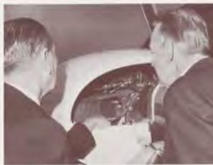
Below —inspector points out frayed cable in engine nacelle to surprised aircraft operator.
