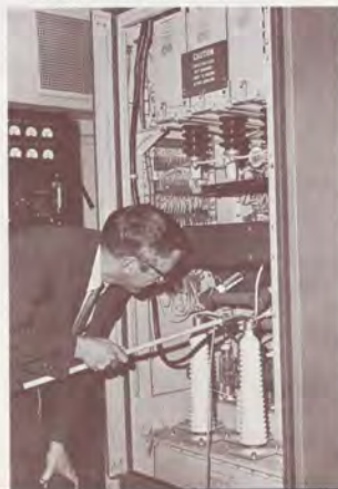
Above—NAVAIDs such as VOR on top of Smokies (alt. 4,242) must be kept functioning regardless of weather. Below—airway sector chief uses grounding stick when working on 24,000-volt TACAN.
