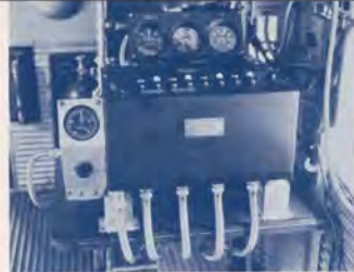
Electronic switching gear designed and constructed by Crane, Holloman and Stout controlled air speed, engine speed, altitude and vertical speed adjustments.
