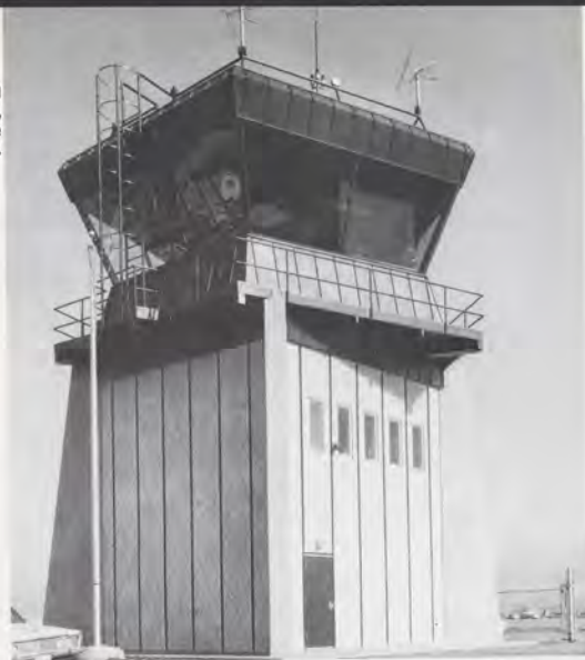
The new compact, transistorized tower at Reid-Hillview Airport, requiring no equipment storage floor, squats close to the ground.
