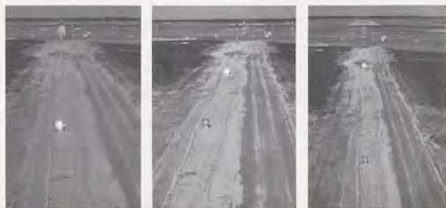
Above—Standard 3,000 foot approach lights mounted on pilings, Washington, D. C. Right—Sequenced runway alignment lights used alone at Atlantic City, N.J. in test of low cost approach lights
