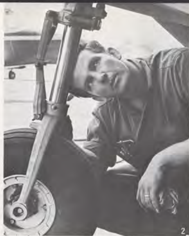
1 Specialist guides prop to bench for inspection. 2 Look into wheelwell for signs of chafing, other signs of wear. 3 The right tool for the job is the sign of a good mechanic, a lesson pilot-owners should learn early. 4 Special fixture speeds job, adds to safety.
