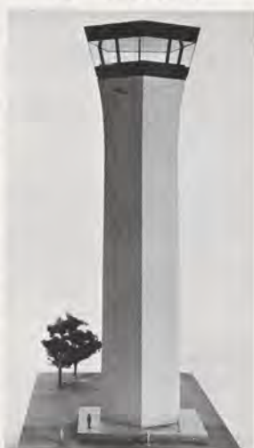
The FAA will receive bids this month for construction of 10 concrete-shaft airport traffic control towers at U. S. airports. All will be of one standard design. Size will depend upon activity.
