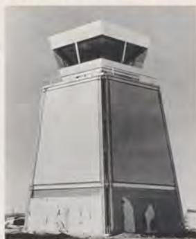
Lawton, Okla., tower while under construction.
