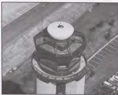
The ASDE-3 Antenna monitors ground traffic enabling air traffic controllers to see positions of aircraft, fuel trucks and other traffic on airport property.
