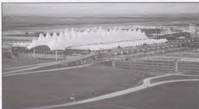
The main terminal building, named after Elrey Jeppesen, a Colorado aviation pioneer, is distinguished by a 34-peak tensile fabric roof.
