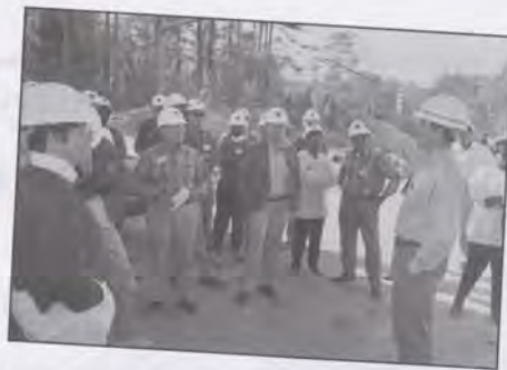
FTA Deputy Administrator Grace Crunican, left, looks on as Resident Engineer Dewey Martin explains the construction techniques used on the MARTA line between the new Medical Center and Dunwoody stations.
