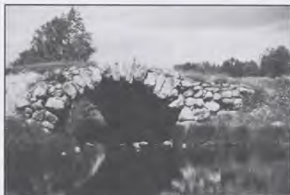
Stone arch bridge, still in service for local traffic near Tver, Russia
