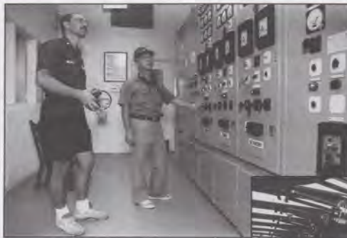
Above: MK3 George Wieland from Loran Station Marcus Island shows a JMSA crewman how to make the station's twin diesel generators parallel - ensuring both are producing the same amount of power. The generators are a vital part of the station. As the only source of power, they keep a radio beacon on air which thousands of mariners and aviators depend on for navigation.
