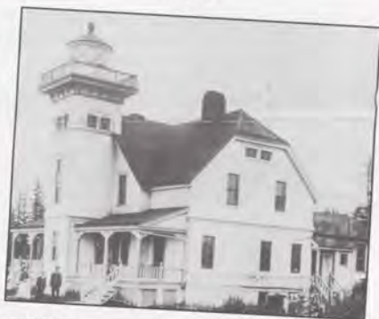
Sentinel Island Light Station, one of the first U.S. built lighthouses in Alaska. Built of wood, it began operating in 1902. Photo courtesy of the Alaska State Historical Library.
