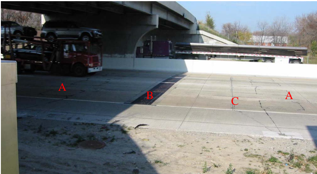
Figure 2.9: Borman Expressway Weigh in Motion
