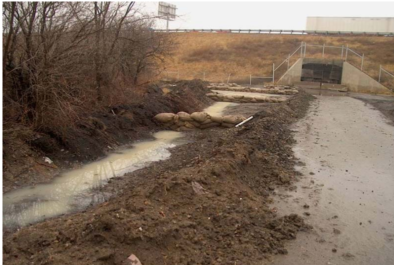
Figure 10. Interstate 65 site in May 2002.
