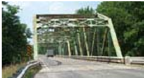
Figure 7. Many INDOT bridges have been painted with lead-based paint.
