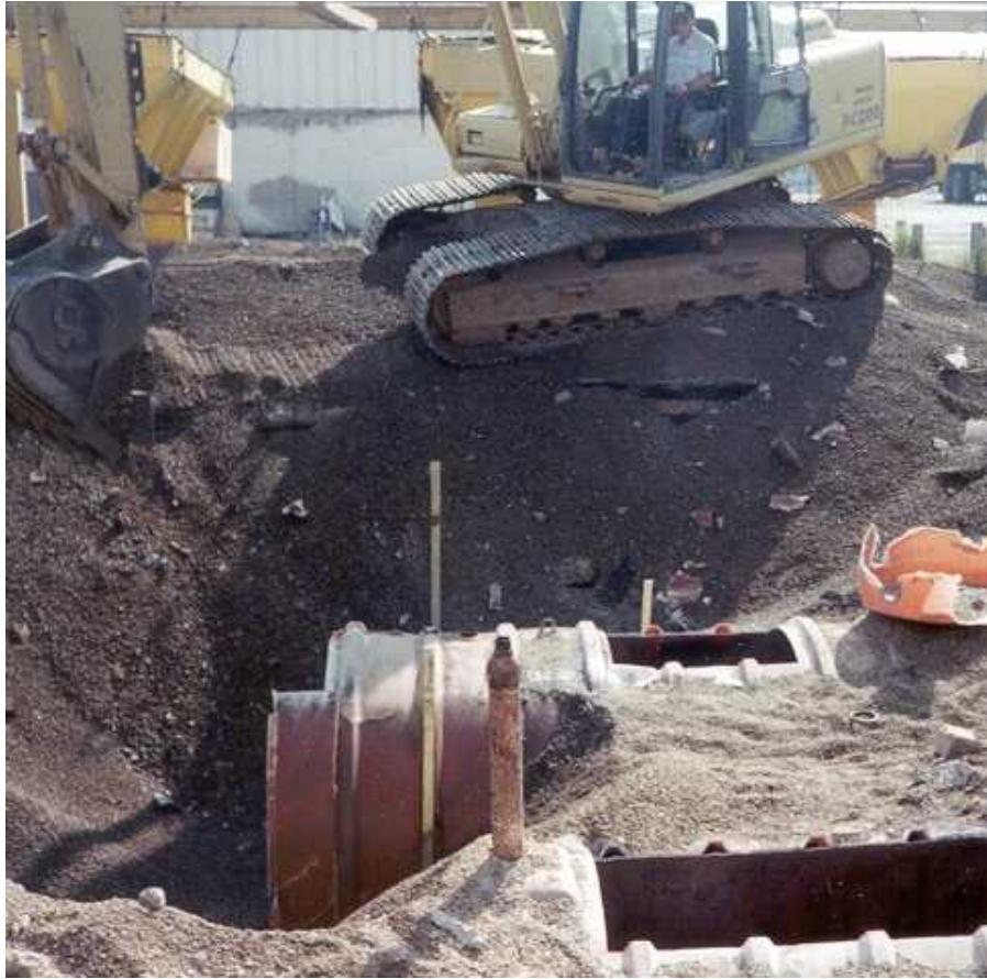
Figure 6. Excavator removing an underground storage tank
