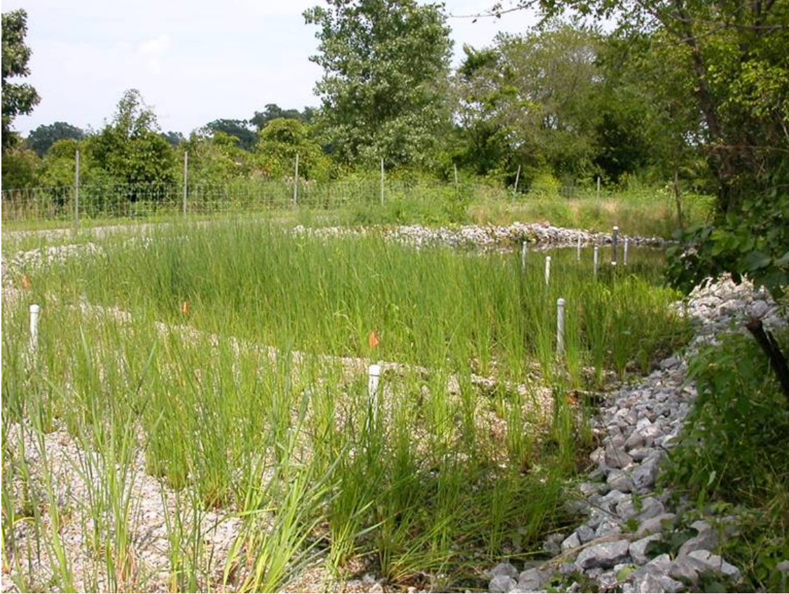
Figure 11. Interstate 65 site in late July 2003 showing the constructed wetlands.
