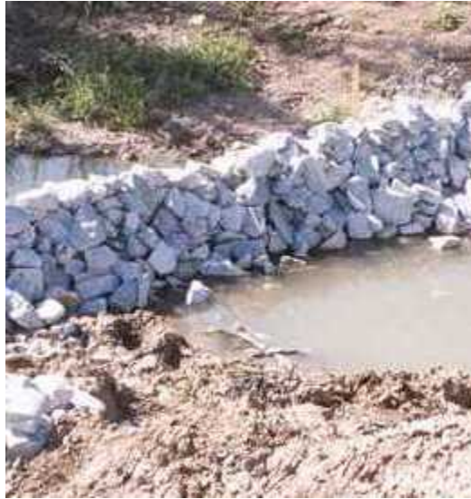
Figure 8. Soil erosion control implemented by INDOT
