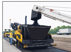
Loading Mixture onto Paver
