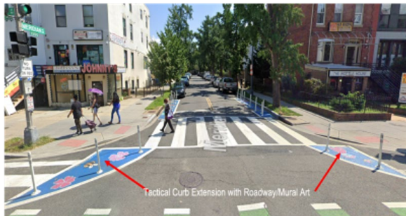
Figure A3 Tactical curb extensions with roadway / mural art (Image Source: Map Data ©2023 Google)
