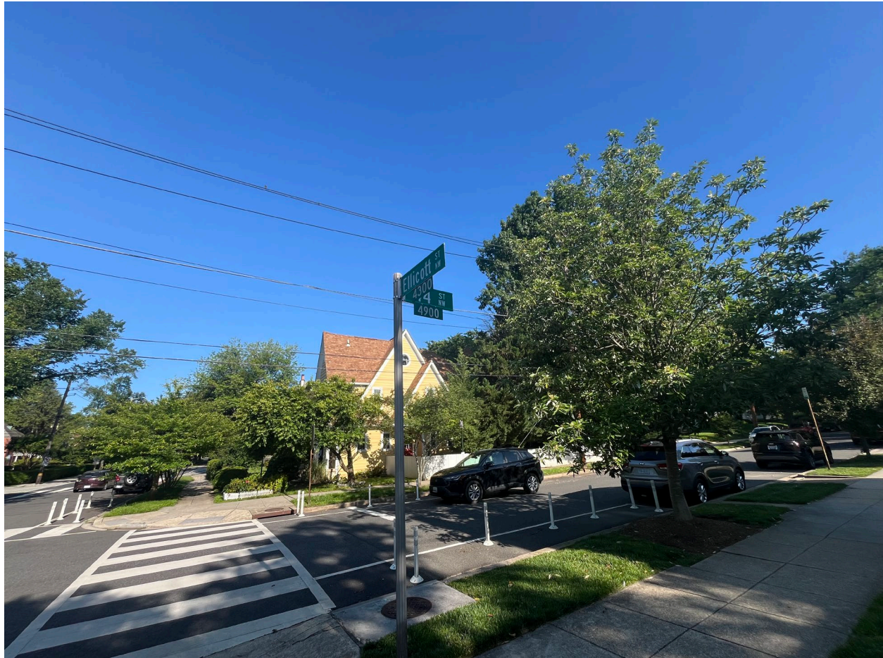
Figure 3-2 A Tactical Curb Extension at 44th St NW and Ellicott St NW
