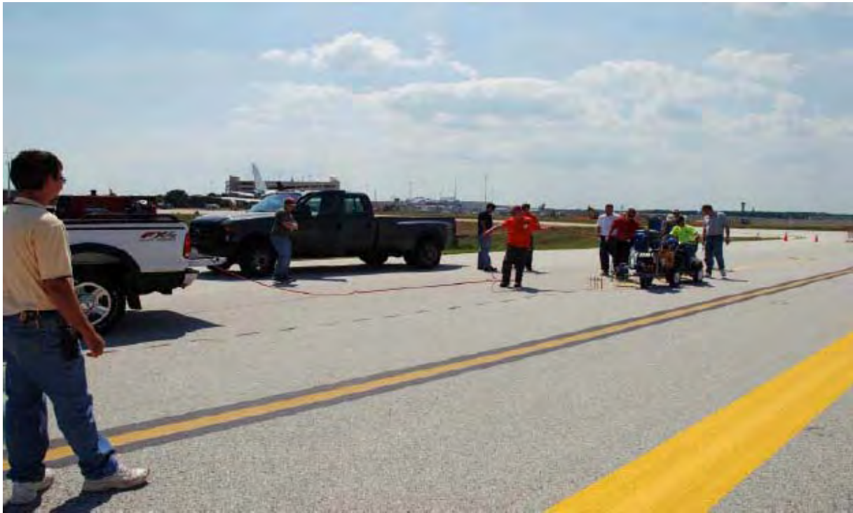
Figure 10. Applying 18" x 150' Friction Lines on Aged HMA at Test Site Three
