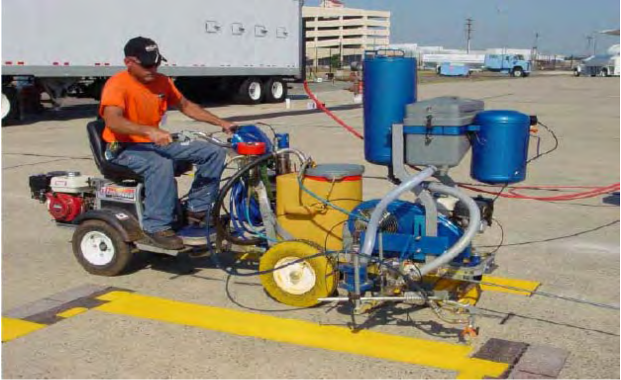
Figure 6. Applying 12" x 6' Edge Lines on Aged PCC at Test Site Two
