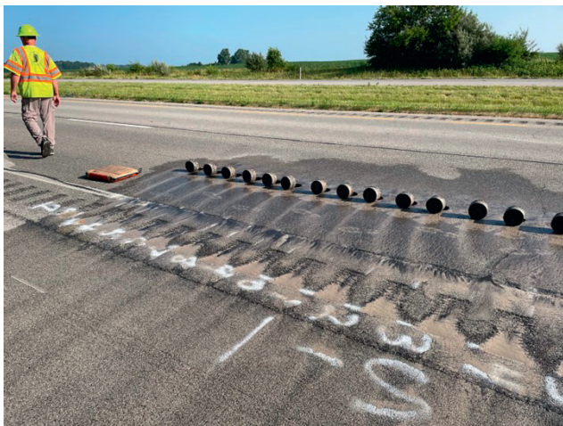
(c) Lane center coring on I-74
