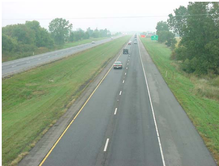
Figure 6-4 Interstate 65 Northbound at 137 th Avenue, Posted Speed Limit 65 mph
