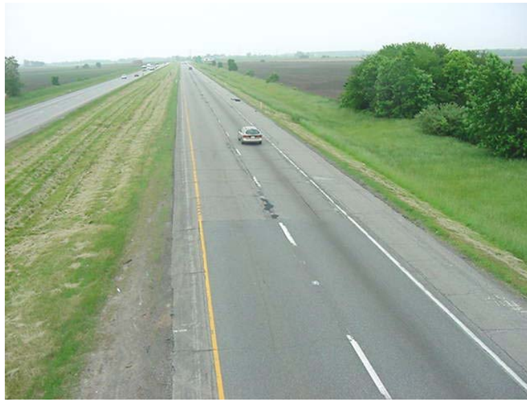
Figure 6-5 Interstate 65 Northbound at 113 th Avenue, Posted Speed Limit 65 mph
