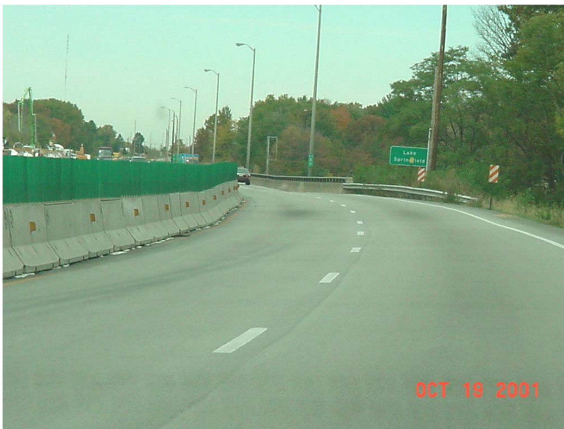
Figure 2-1 Roadway conditions of I-55 during reconstruction of Lake Springfield Bridges(10/19/01)
