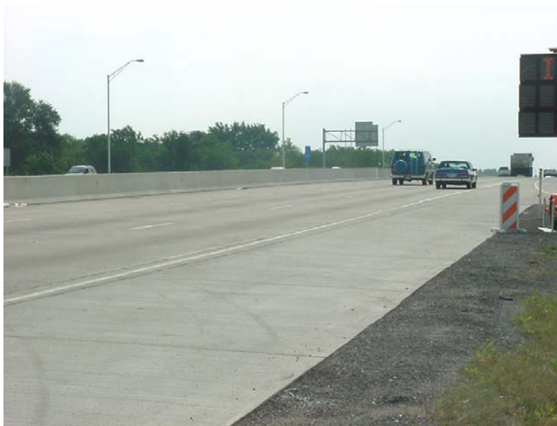
Figure 6-9 Interstate 65 Southbound at Ridge Road
