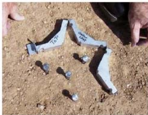
Fig. 5.2 Remove Template to Expose Spikes
