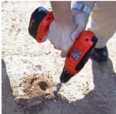
Fig. 5.6 Remove Soil with Power Drill
