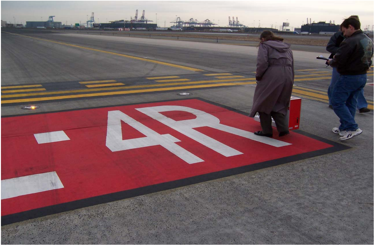
Figure 14. Thermoplastic Marking Material After 6 Months at EWR
