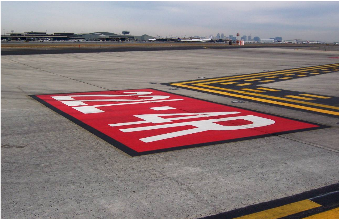
Figure 12. Thermoplastic Runway Identification Marking at EWR
