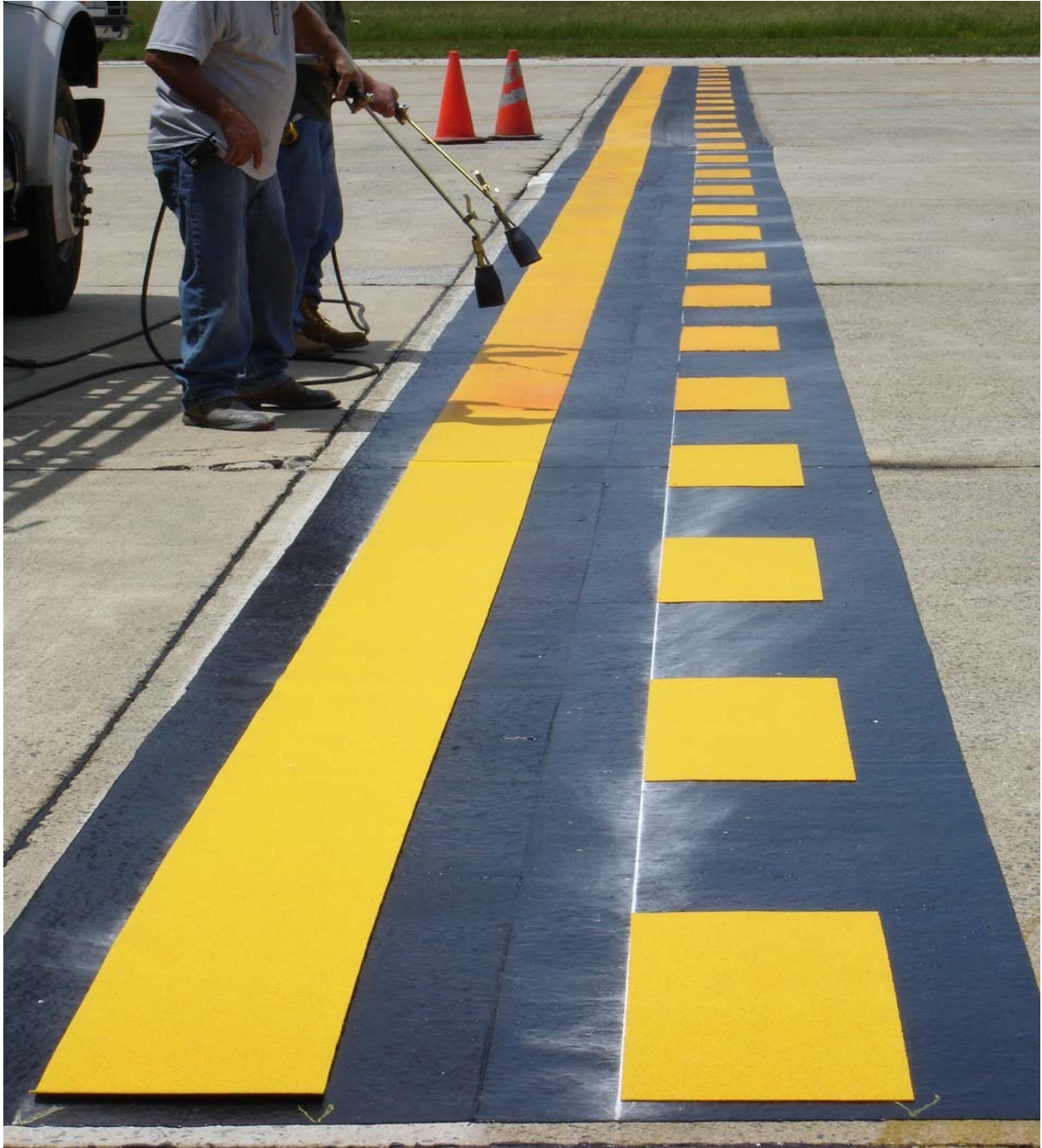
Figure 1. Movement/Nonmovement Line on PCC at FAA William J. Hughes Technical Center
