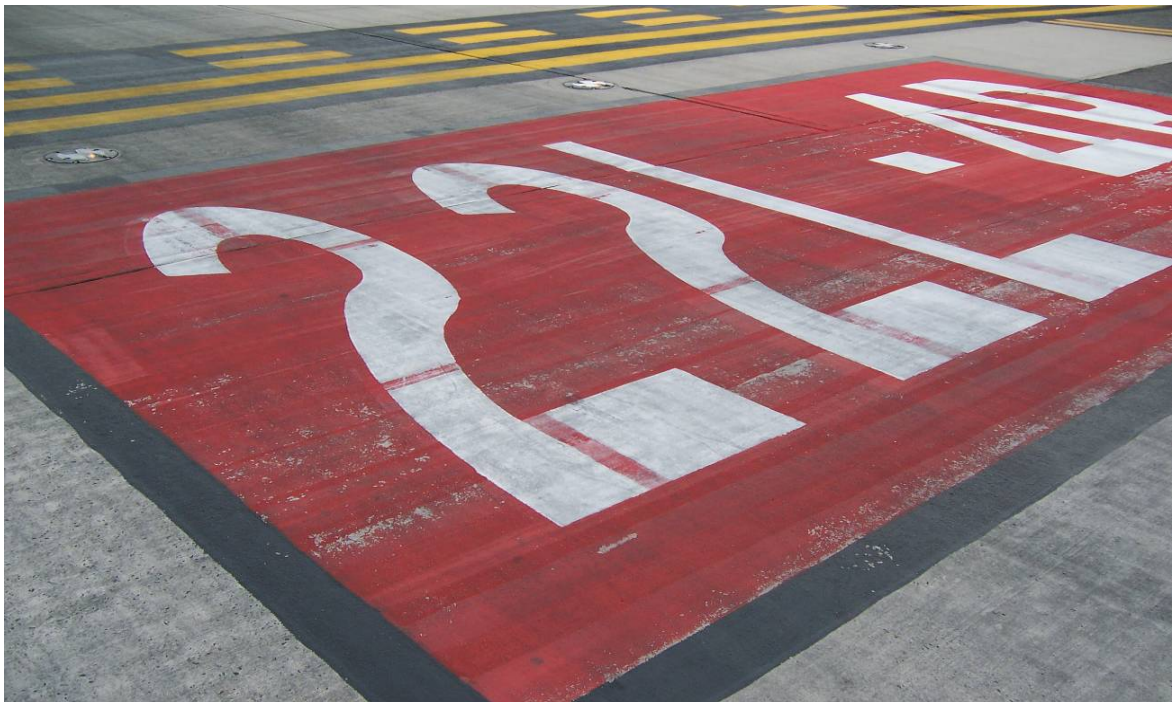
Figure 15. Standard Waterborne Paint After 6 Months at EWR
