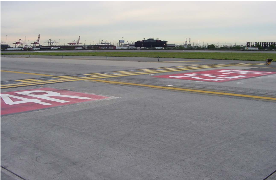
Figure 8. Side-by-Side Markings at EWR
