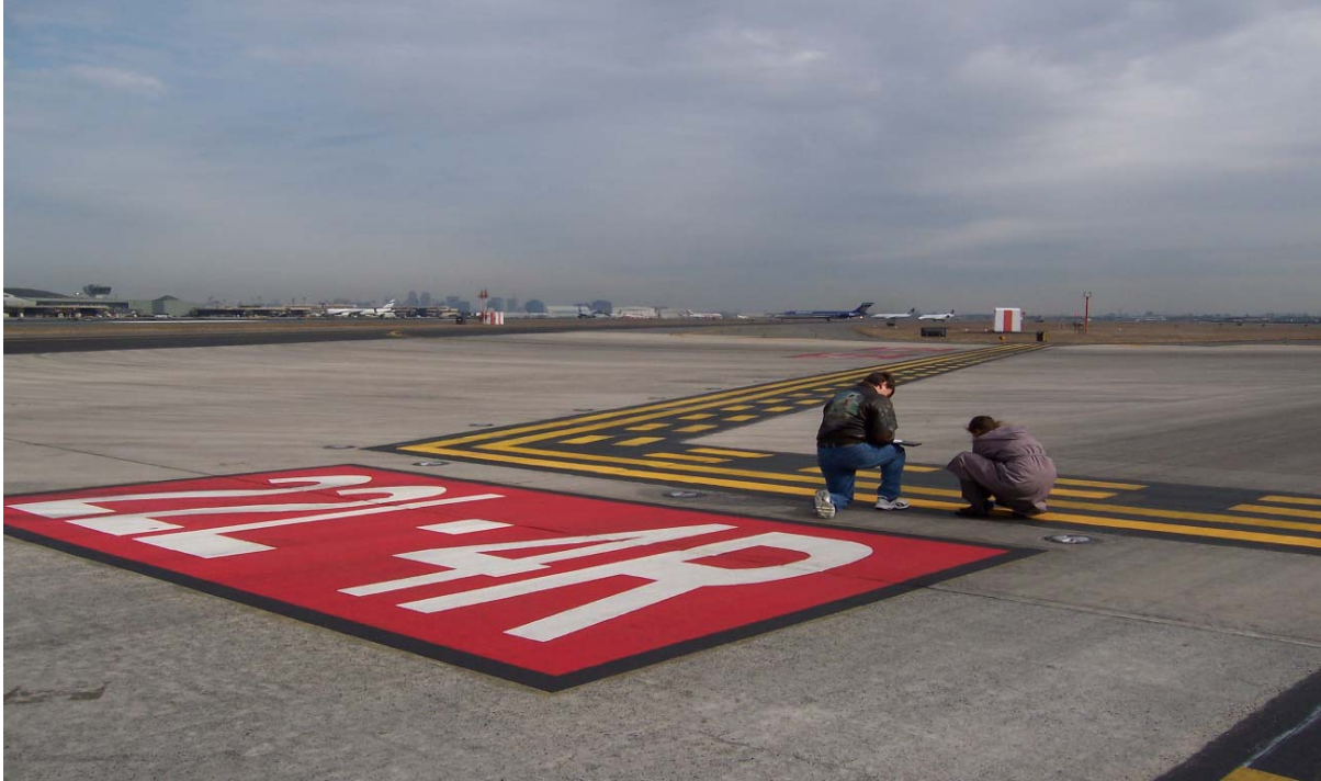
Figure 9. Thermoplastic Runway Identification Marking and One Solid Yellow Line of the Runway Holding Position Marking
