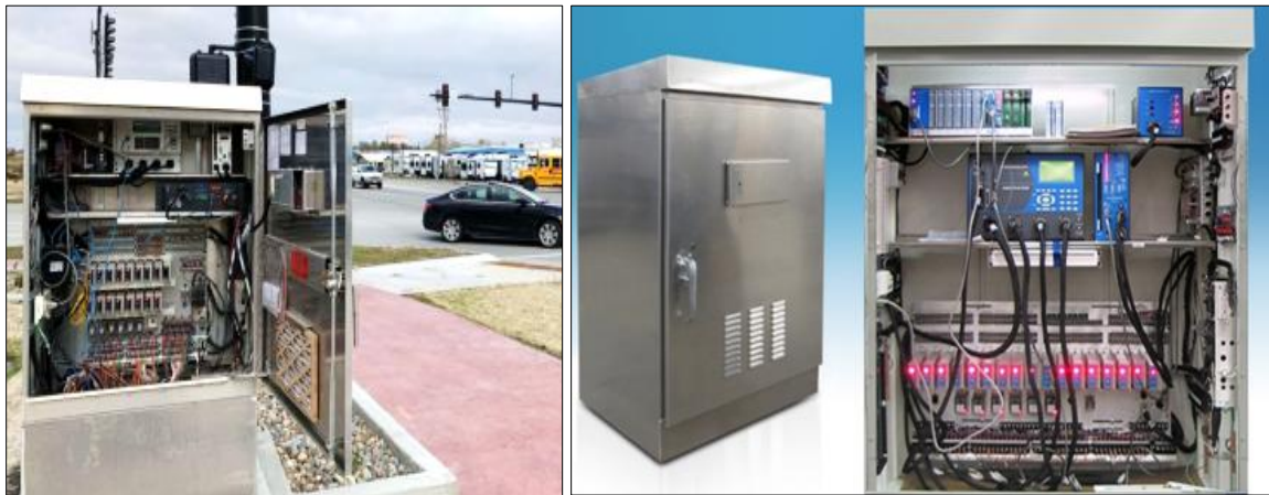
Figure 2.1: Typical TSC system
