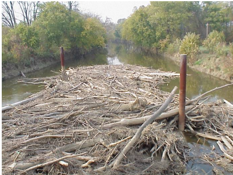
Figure 1.2: View of the Eel River site from bridge deck in upstream direction: a) site cleared of debris (April 2001), b) site with debris pile after a major flow event (August 2000); cylindrical vertical structures are debris deflectors
