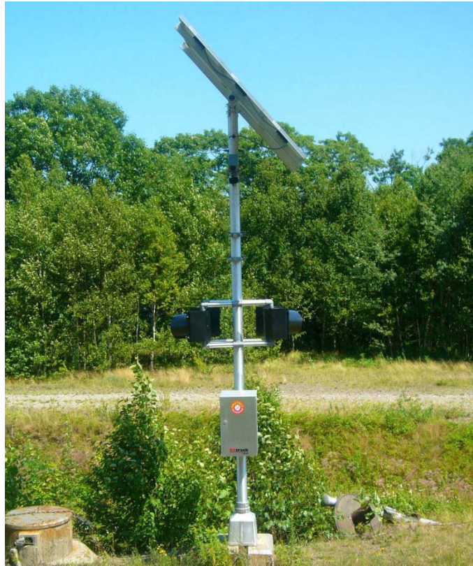
Figure 7. TC Low-Cost Warning Device Configuration (Hildebrand, Roberts, and Robichaud, 2007)
