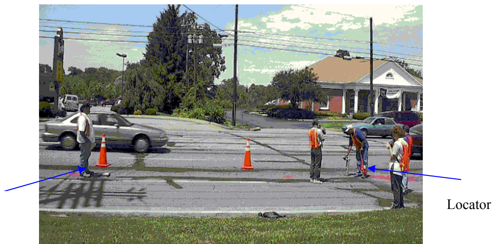
Figure 7.25. Applications of Pipe and Cable Locator –Inductive Mode
