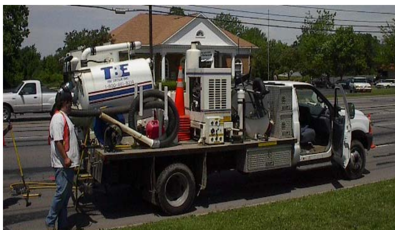
Figure 5.32. Self-contained Vacuum Excavation Truck Systems
