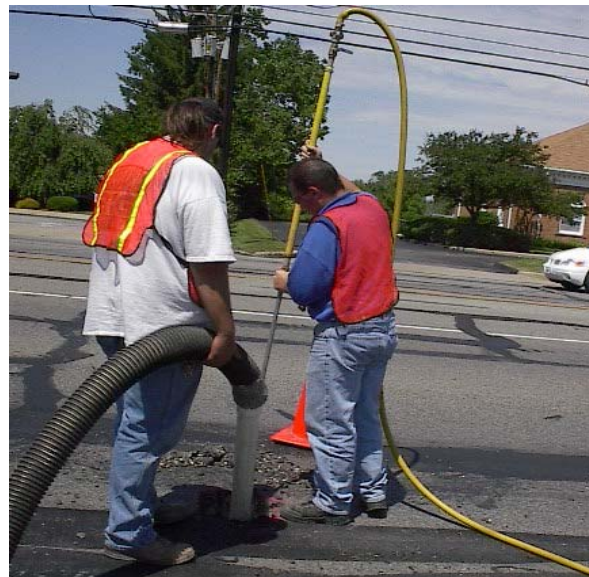
Figure 5.31. Reduction process with High-Pressure Air
