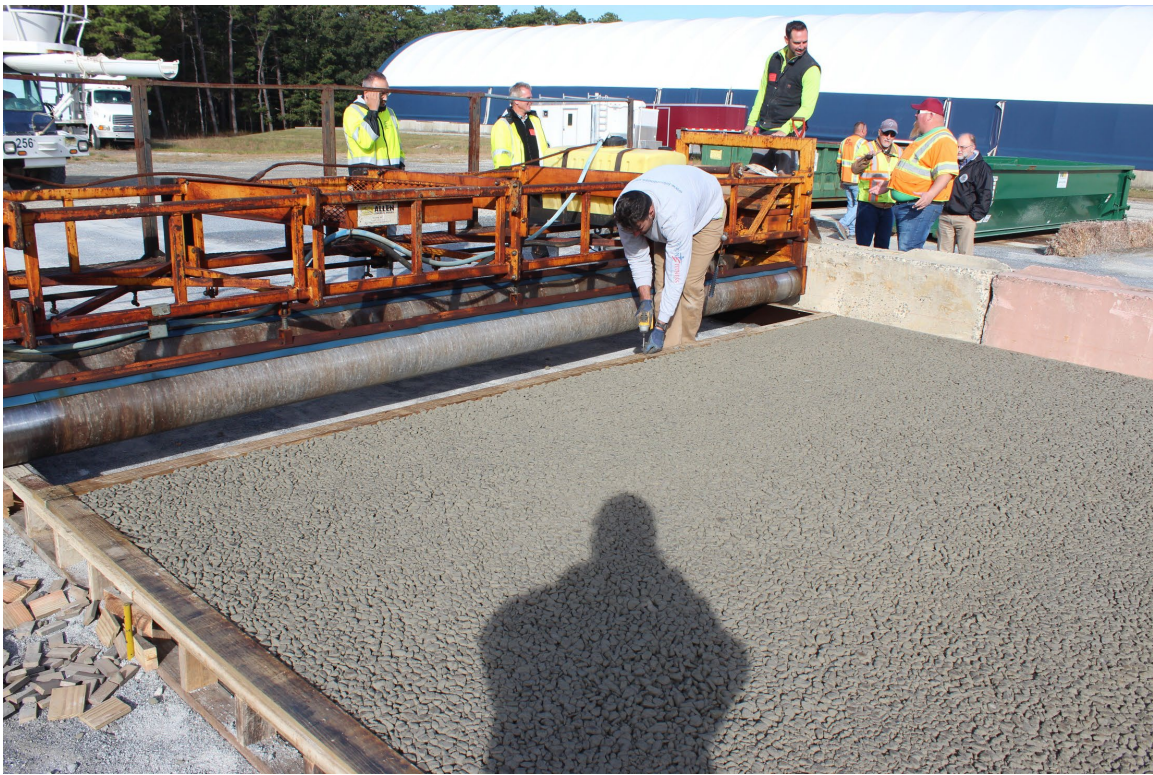
Figure 4. Removing Forms from the Third CTPB Test Strip, October 11, 2019
