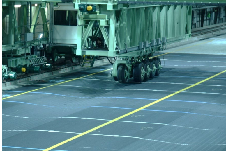
Figure 21. Deformed Surface of the CTPB Test Item After 40,920 Passes (November 3, 2022)
