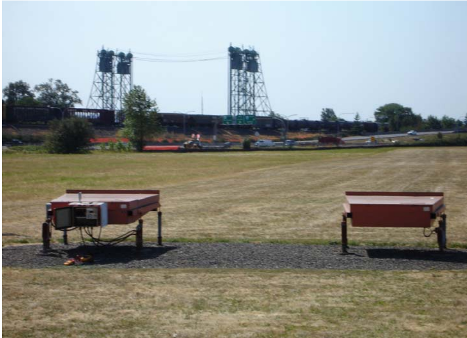
Figure B-1. Interstate I-5 Bridge Forming Obstruction
