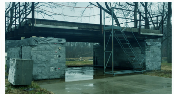
Source: FHWA. Test specimens from a decommissioned bridge.
