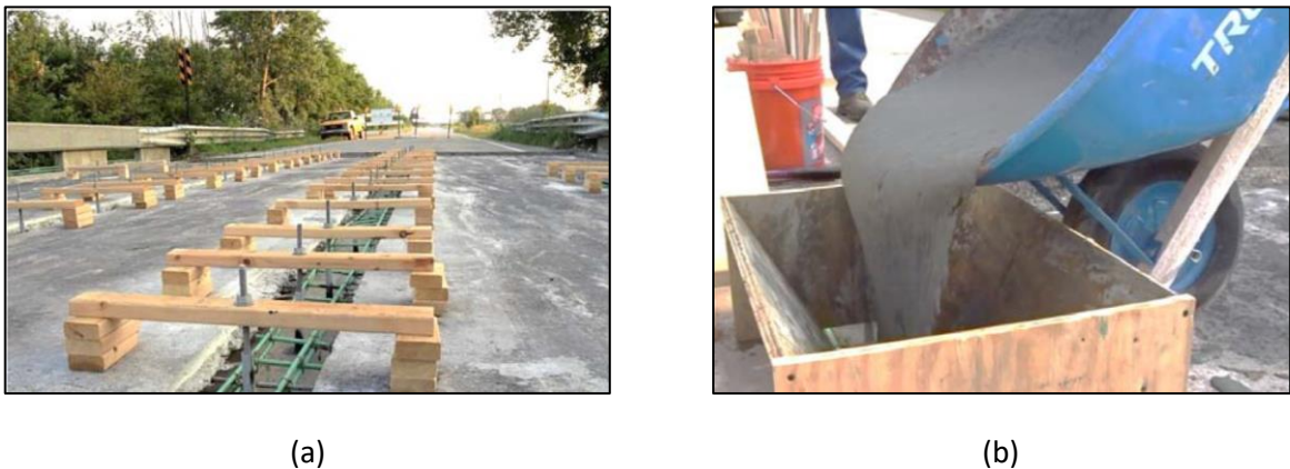
Figure 2.23 (a) Closure pour, and (b) UPHC placement (Michigan DOT 2018).
