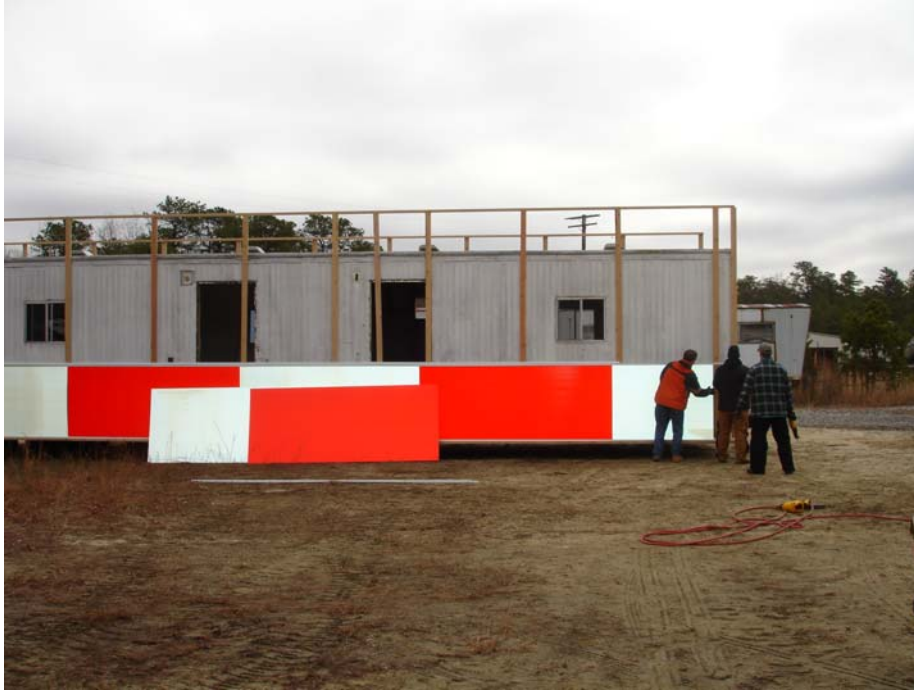
Figure A-1. Construction
