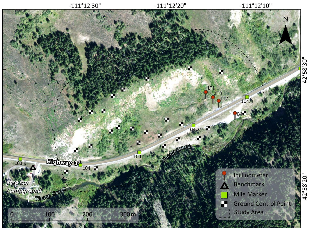
Figure 3.36 Pine Bar Landslide Area along US 36 in Caribou County Idaho
