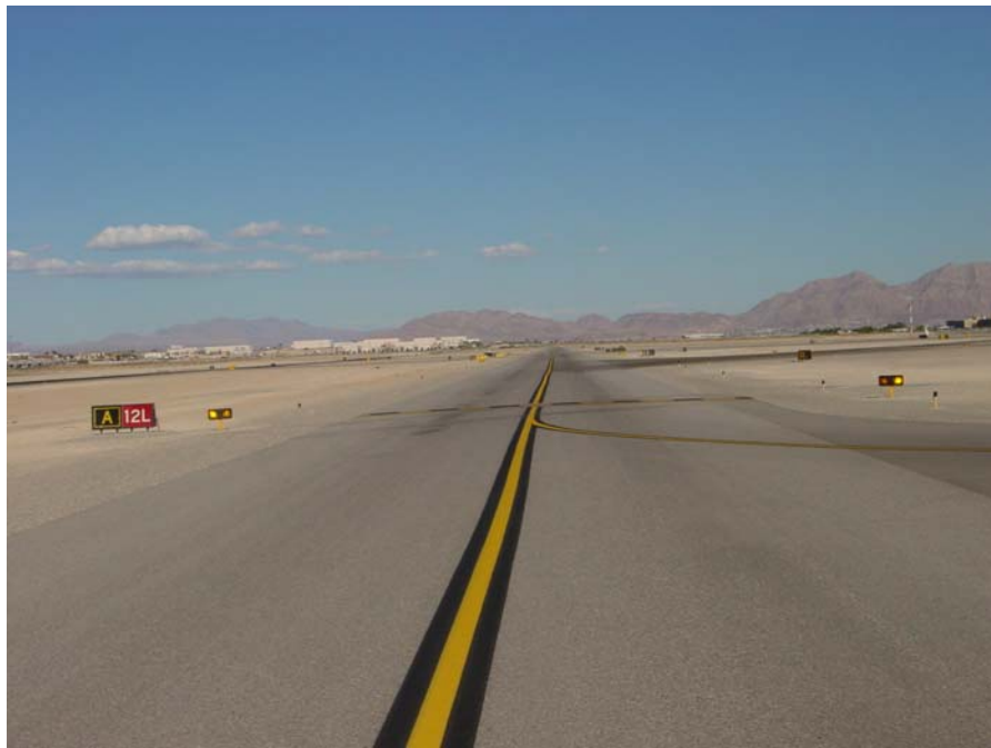
Figure A-8. Alpha 4—Runway 12L-30R and Taxiway A (West side)
