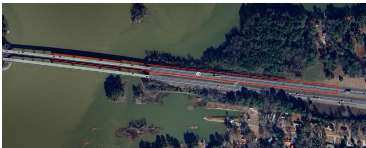
Figure 3-9 Work Zone (Merge) Field Data Collection Location (I-20, Lincoln, AL)
