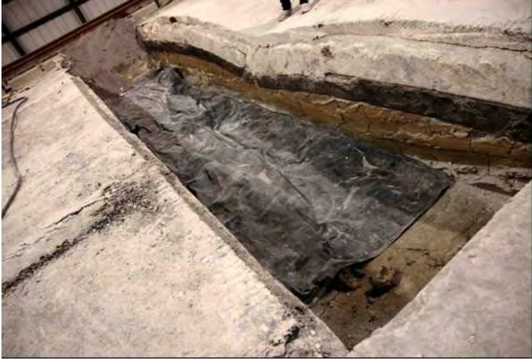
Figure 26. The MRC-E Trench
