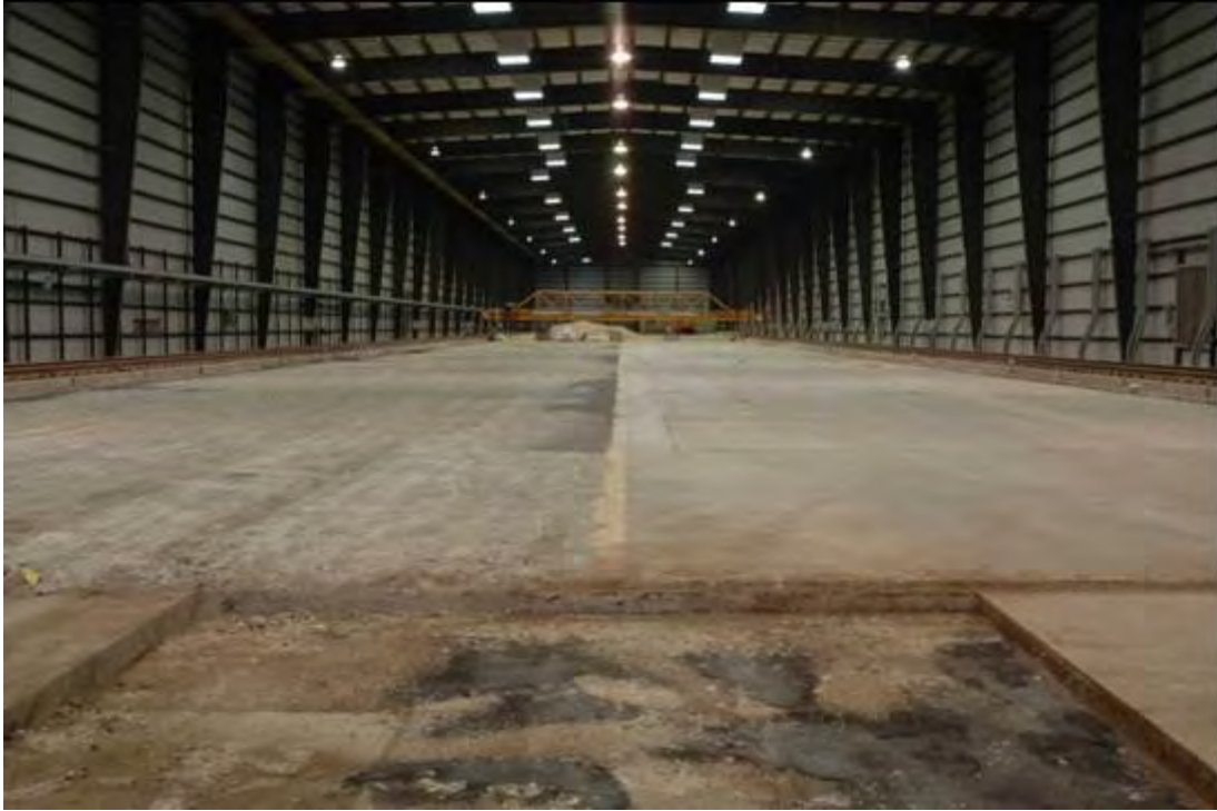
Figure 4. Rubblized on the Left (North), Nonrubblized on the Right (South)
