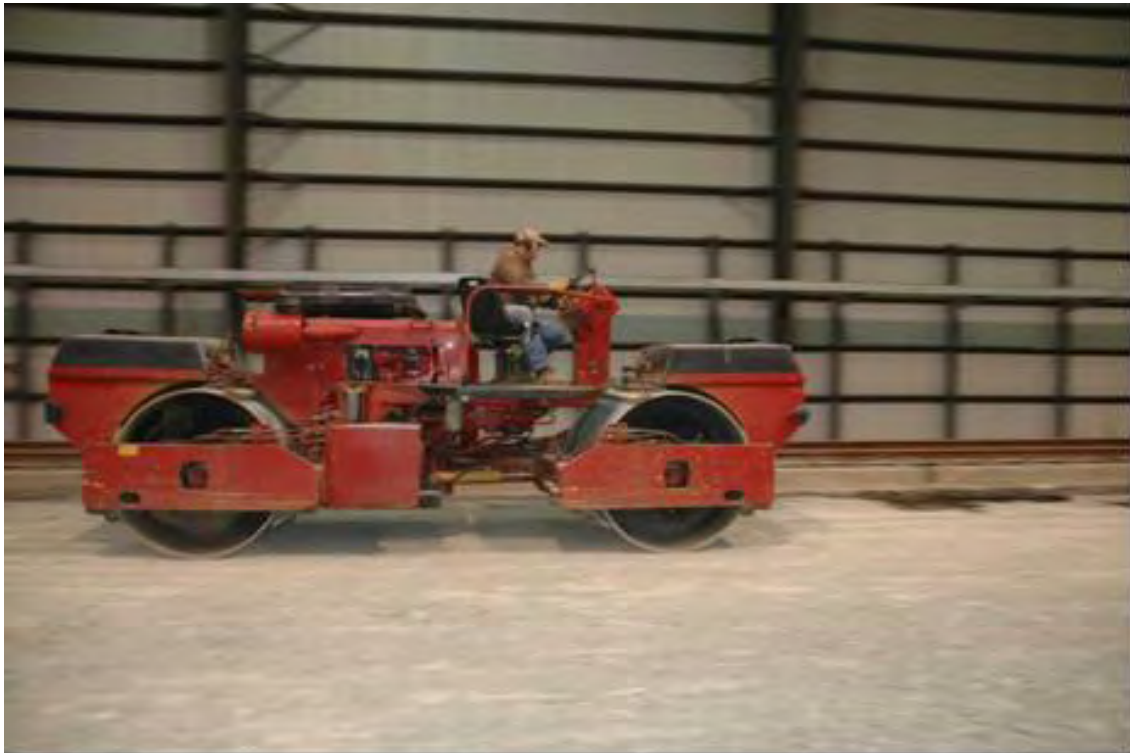
Figure 3. Rolling the Rubblized Pavement
