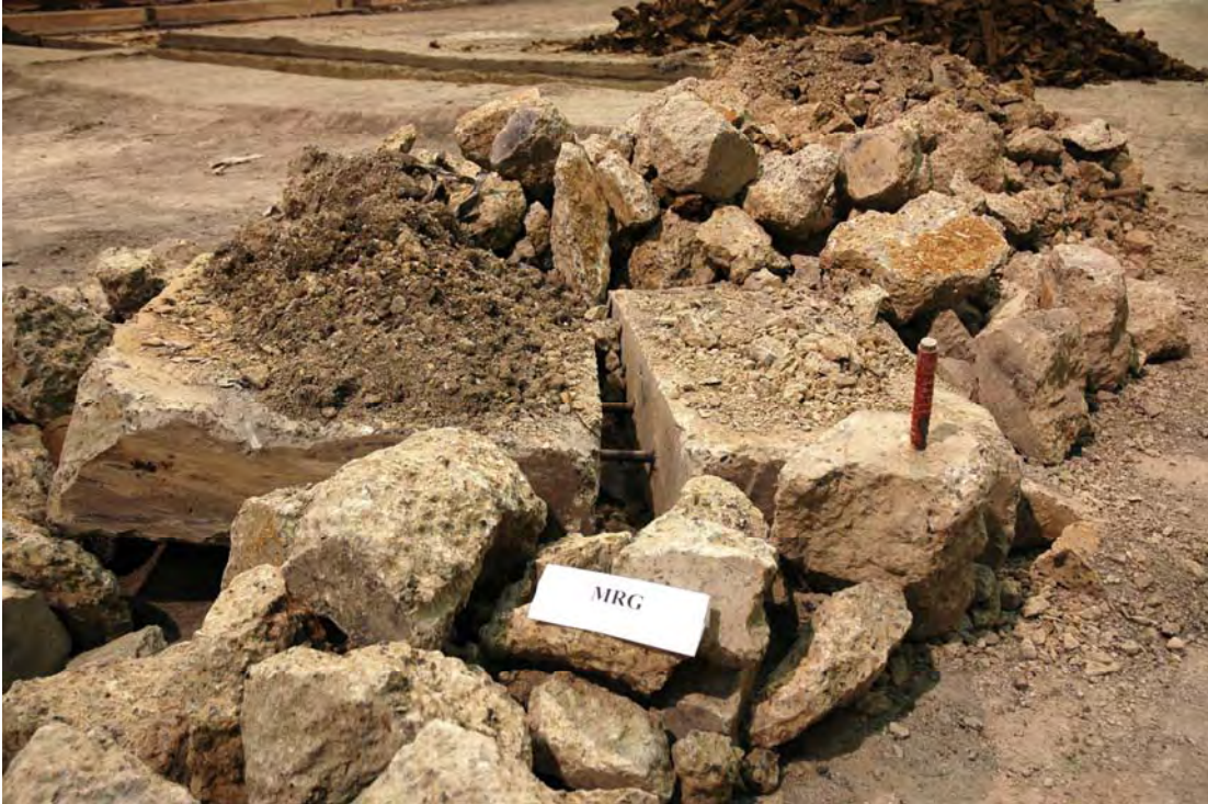
Figure 35. Rubblized Concrete Pieces Still Connected With Dowels
