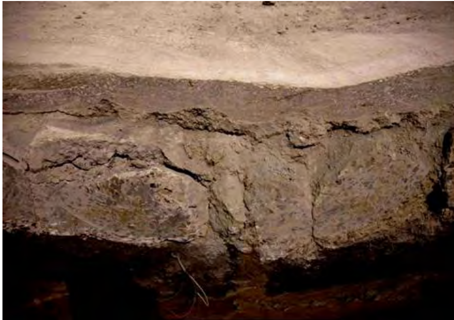
Figure 25. Close-Up of Failure Zone (MRC-W)
