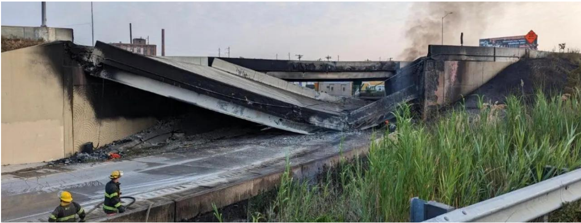
Figure 2-2: Illustrations. Images for the June 2023 tanker fire at the Cottman Avenue exit ramp underneath I-95 in Philadelphia, PA: (a) roadway plan view and (b) photo of the aftermath of the fire event [19].
