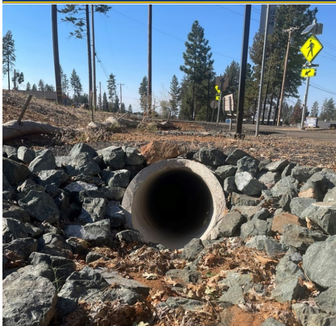
Figure 14. Photo. Concrete culvert pipe in Paradise, replacing an HDPE pipe.
