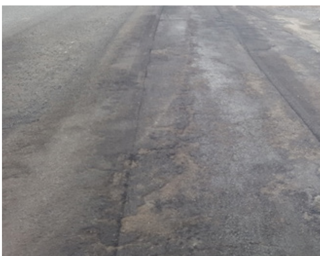
A. Delamination.
