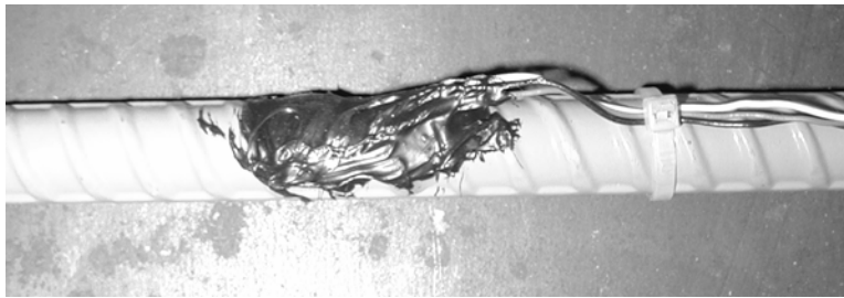
Figure D.3: Applied Strain Gage Protected with M-Coat J
