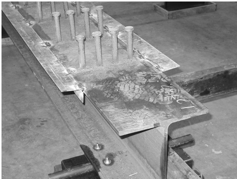
Figure 4.6: Cold-Rolled Angles Welded to Top Flange of Girder
