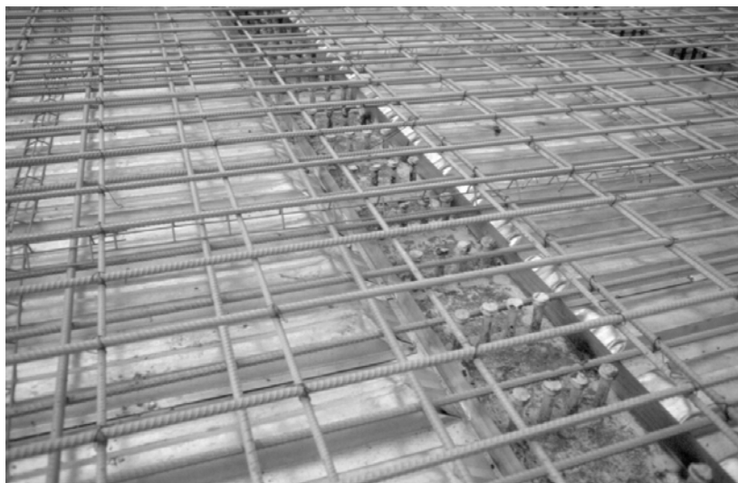
Figure 3.10: Reinforcement in Positive Moment Region
