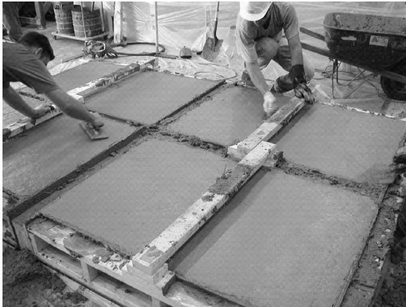
Figure 5.27: Deck Model Finishing
