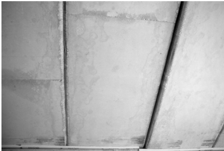
Figure 2.13: Elevation Difference in Box Girders (Bridge 14)
