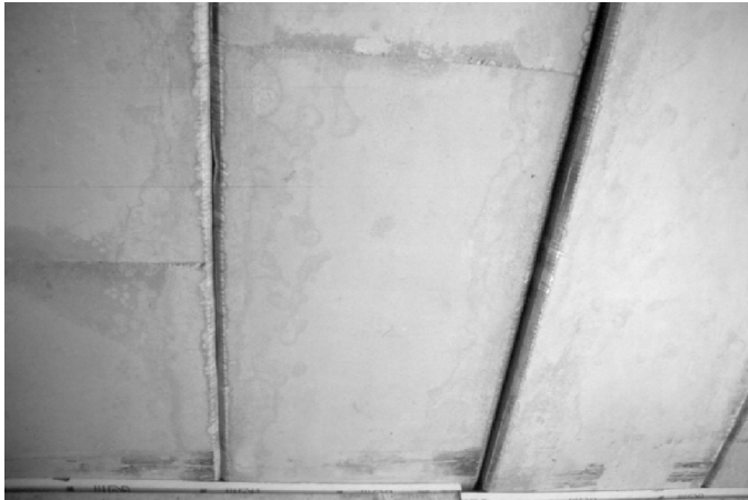
Figure A.14.3: Elevation Difference in Box Girders
