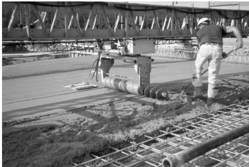
Figure 3.13: Mechanical Screeding of Deck
