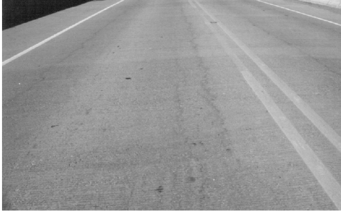
Figure A.17.3: Longitudinal Cracks in Bridge
