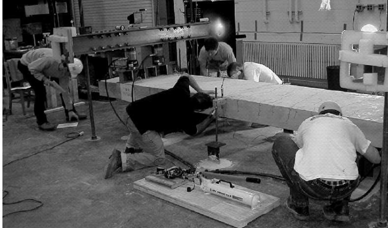
Figure 6.21: Marking Cracks During Testing (Specimen B-9)
