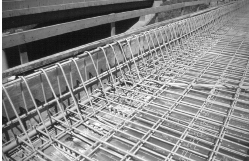
Figure 3.28: PVC Conduit between Mats of Steel in Deck
