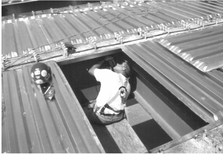
Figure 3.24: Strain Gage Installation on Girder
