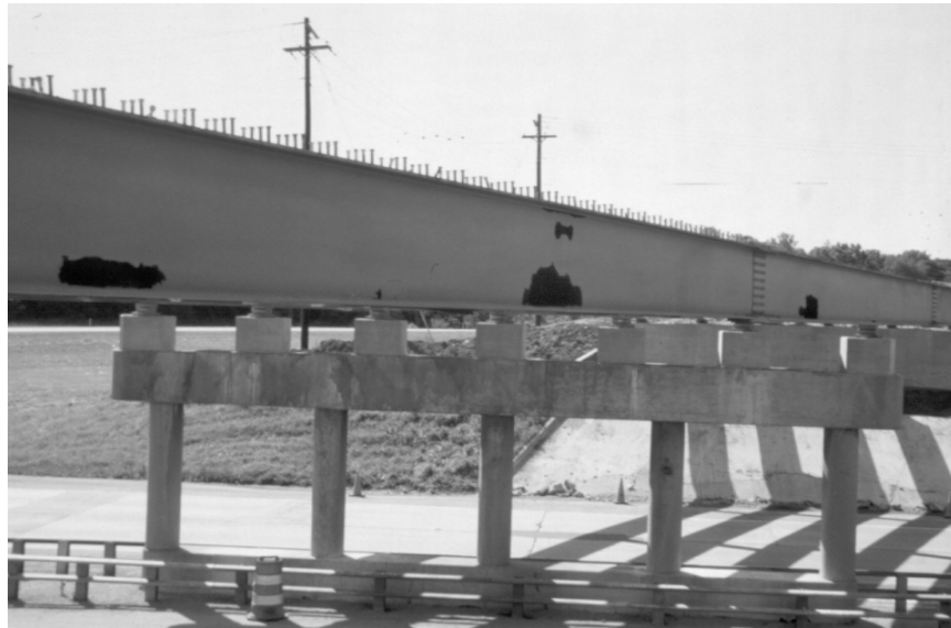
Figure 3.2: Pedestals on Center Pier to Raise Elevation
