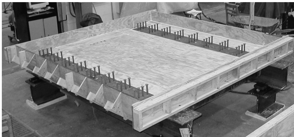
Figure 4.14: Completed Formwork for Free-Shrinkage Model
