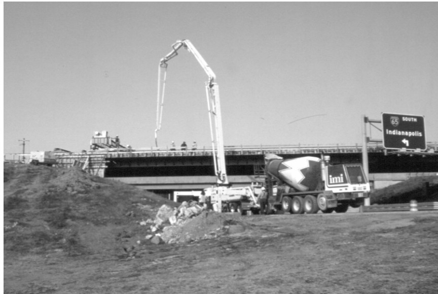
Figure 3.12: Concrete Placement on Deck with Concrete Pump
