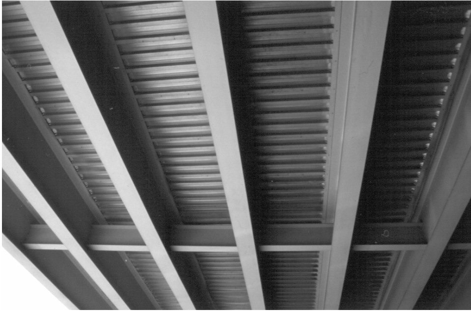
Figure 2.2: Steel I-Beam Superstructure with Stay-in-Place Forms (Bridge 3)
