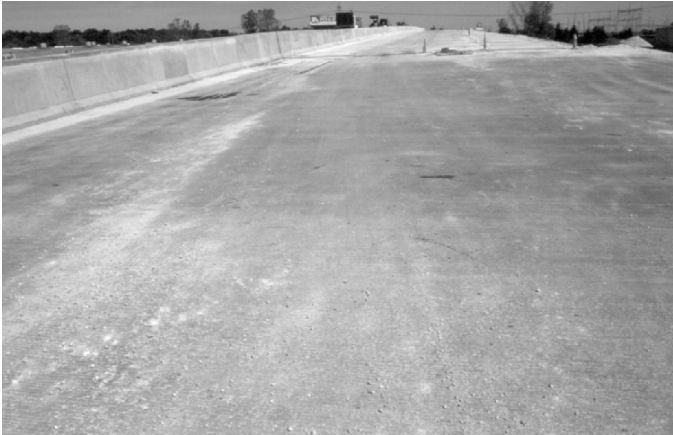
Figure A.13.3: Bridge under Construction
