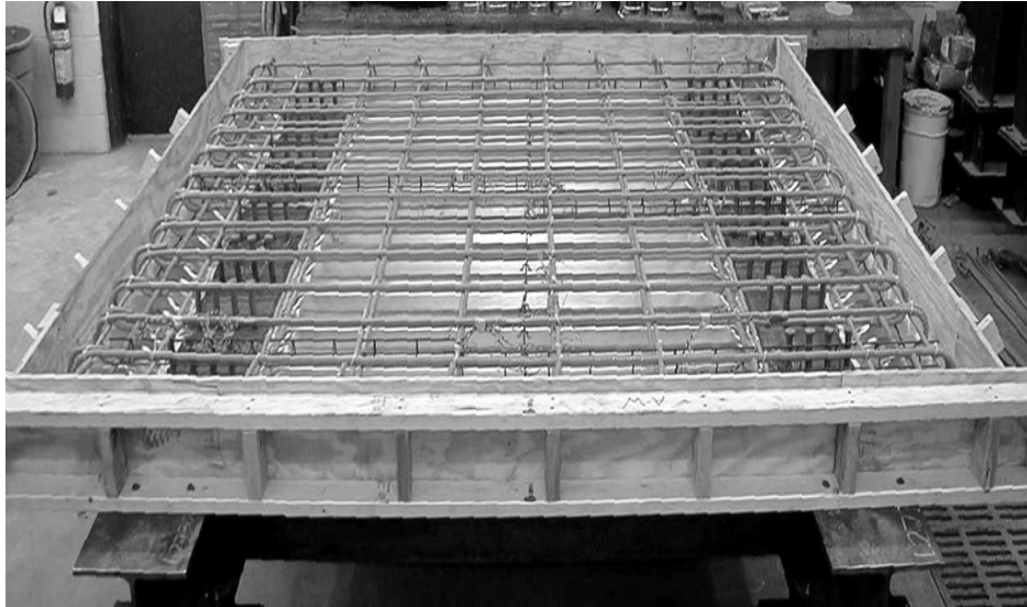
Figure 4.19: As-Built Model with Reinforcement
