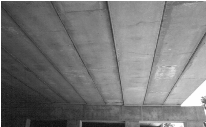
Figure A.14.2: Precast Concrete Box Girder Superstructure
