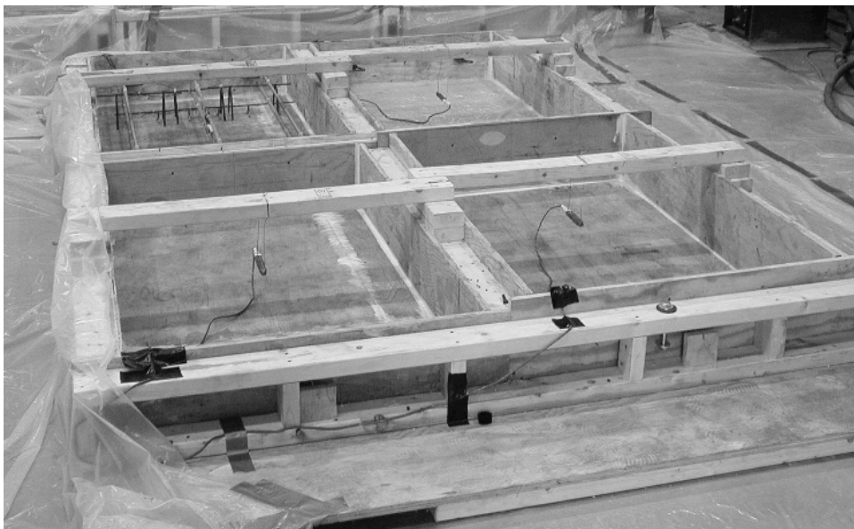
Figure 5.13: Formwork for Specimens 7-10
