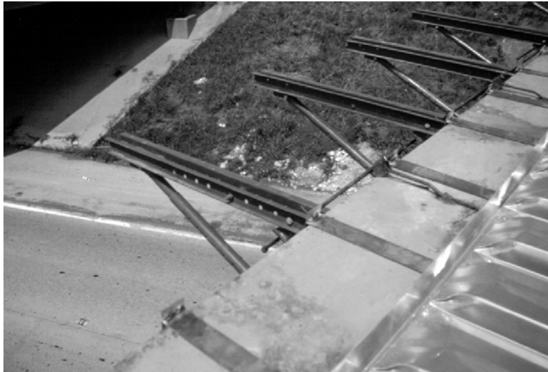
Figure 3.7: Standoffs Attached to Outside Girder
