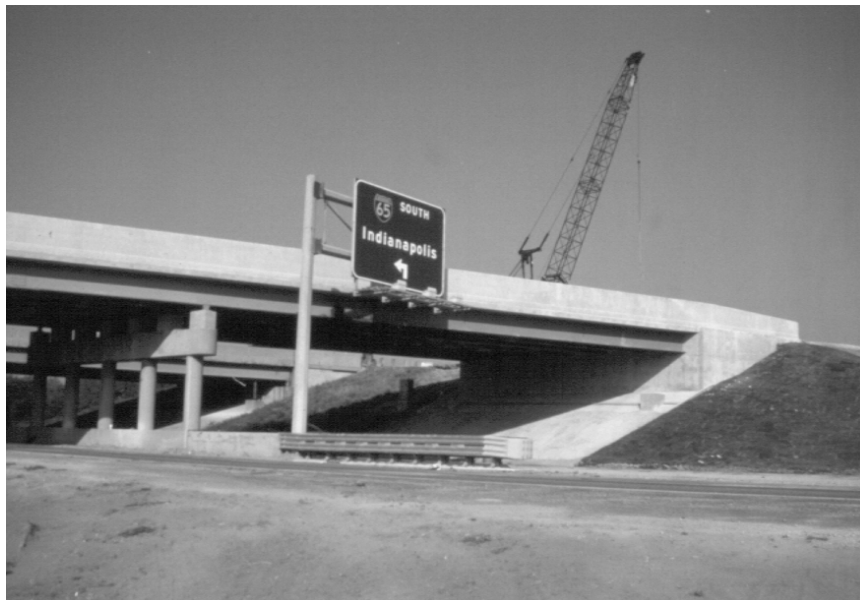
Figure 3.1: Elevation of I65 over SR 25 Bridge
