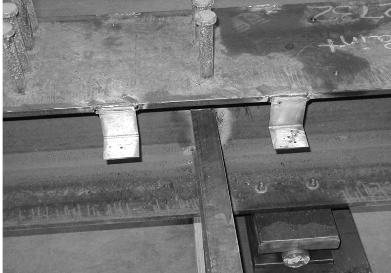
Figure 4.10: Clips Welded to Top Flange of Girder
