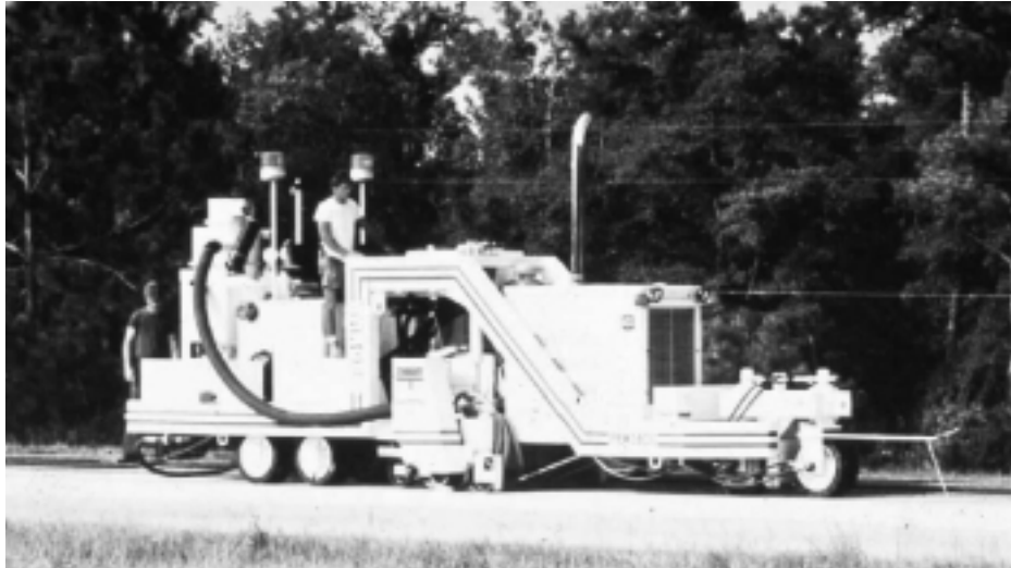
Figure 3-9: Diamond Grinding Operation [Correa and Wong, 1997]
