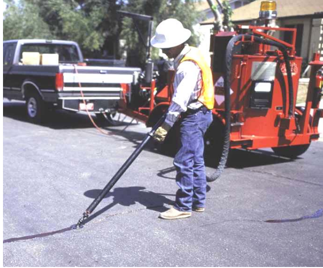
Figure 3-5: Crack Sealing at Sub-district Level in Indiana
