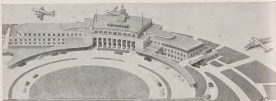
Landward facade of terminal building as shown by architects' model. Spectators enter building from main traffic circle over bridges to the right and left.
