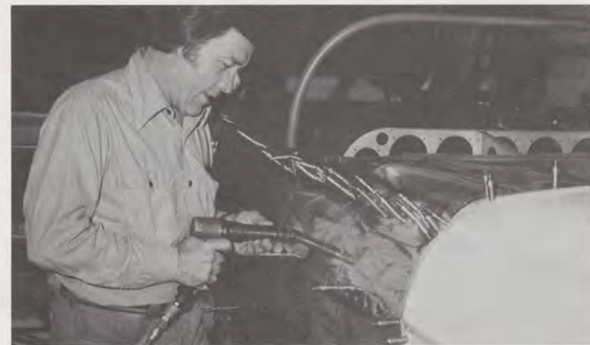
Above: Every component of Pieper's plane has been cut, fitted and assembled by him. Below: Perforated metal plate is a speed brake, just like those on fighter planes.
