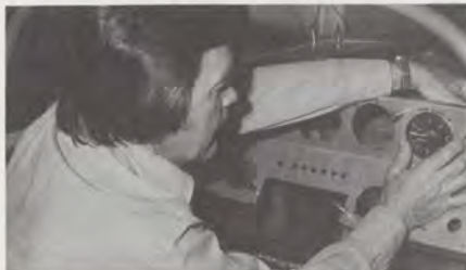
Above: Hanging the engine is a major milestone for amateur aircraft builders. Engine and propeller are second-hand. Left: The instrument panel will be unusually complete, containing some instruments usually found only in planes intended for all weather flight.
