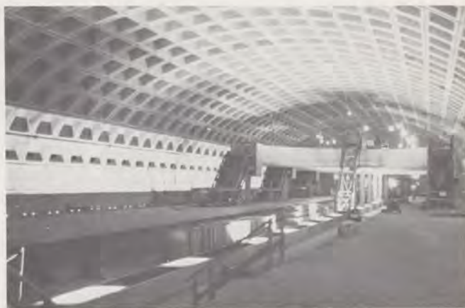
The Metro station serving the Nassif building is 90 feet below the plaza level. Access will be way of an escalator on D Street. In common with the others in the system, the passenger platforms are 600 feet long, ample room to sight your station and to board and debark from the trains in safety.
