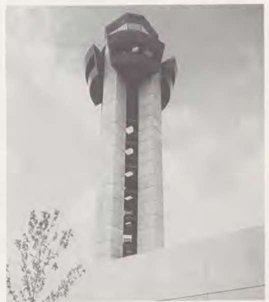
This is the new $7 million FAA control tower at Hartsfield Atlanta International Airport which was dedicated on September 27 by FAA Southern Region Director Phil Swatek. The new tower is 225 feet high and is topped by an eight-sided glass-enclosed cab which has 525 square feet of floor space. A two-story base building contains some 25,000 additional square feet housing the terminal radar control (TACON), administrative offices, and training rooms.
