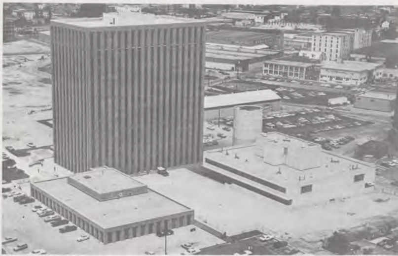
DOT's Transportation Systems Center is located at Cambridge, Mass., a five-minute rapid transit ride from historic Boston Common. Acquired from the National Aeronautics and Space Administration in 1970, the $40 million, six-building complex is completely equipped to perform multi-modal research and development.
