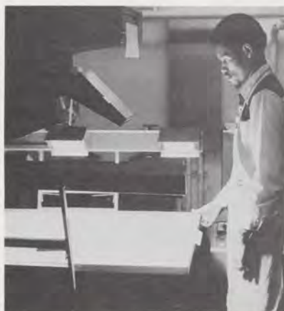
John D. Butler operating an Itek electrostatic plate maker in the P-2 level print shop. The plates will then be used on the small offset presses. Dorothy Jenkins is stripping "flats", which contain photo negatives, in preparation for using them to make metal printing plates for the Harris press.
