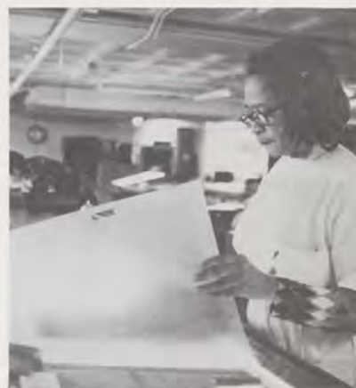
John D. Butler operating an Itek electrostatic plate maker in the P-2 level print shop. The plates will then be used on the small offset presses. Dorothy Jenkins is stripping "flats", which contain photo negatives, in preparation for using them to make metal printing plates for the Harris press.
