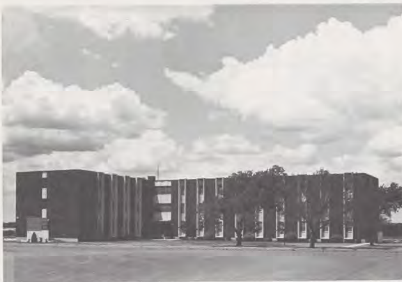
This is the FAA building on the Cameron College campus, some 90 miles south of Oklahoma City, Okla. It houses the management training school offices, seven classrooms and associated conference rooms, and an electronic maintenance room for FAA equipment. The classrooms are within 200 yards of the dormitories, dining room and student lounge.
