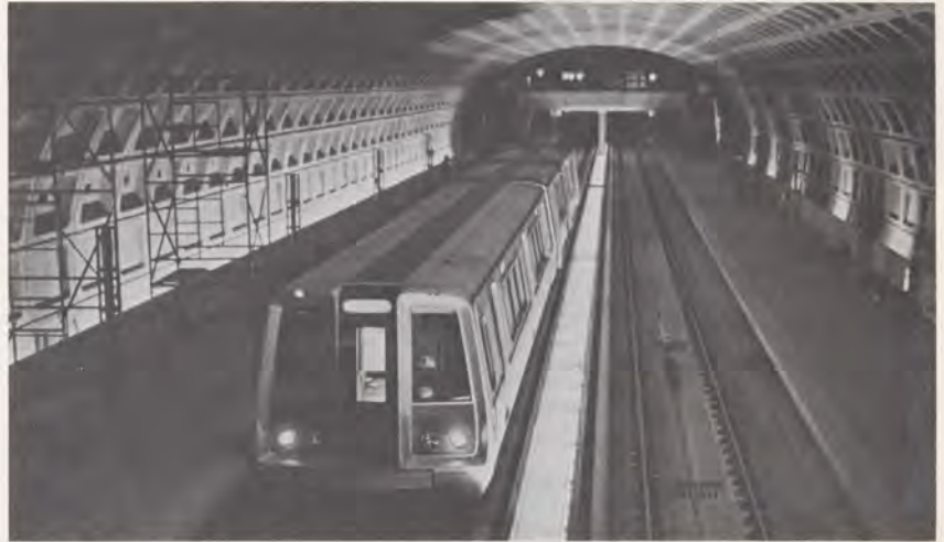
The L'Enfant Plaza Metro Station serving DOT headquarters will look like this one at Judiciary Square. Cars travel east-west in center lanes and passengers enter and leave via broad walks on both sides. Trains running north-south under 7th Street pass through the station along both sides of the tunnel, with the passenger walk in the center.
