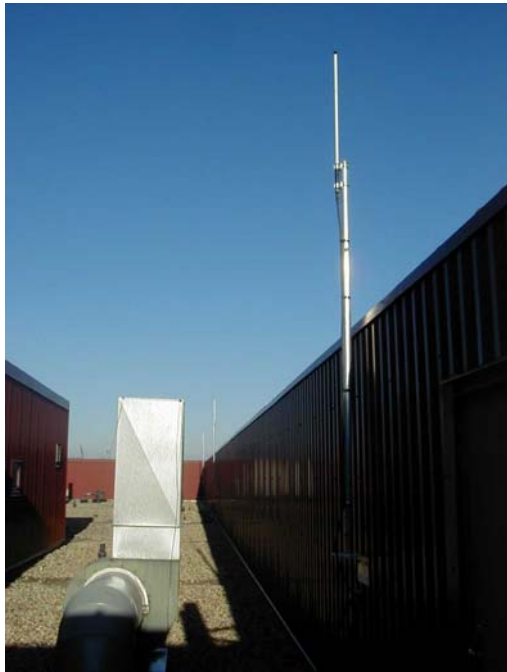
Figure D-2: (Top) View of MSEE building showing three testbed antennas over the roof-line. (Bottom) View of testbed antennas from on the MSEE roof.
